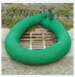
Inlet Protection: SiltSoxx can be used around drain inlets, in front of curb inlets, and as a curb sediment containment system.
